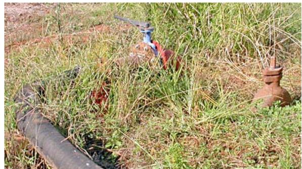
Permanent pipe with valve and connection to flexible pipe to pump. The valve and connection can be seen to the left of the pump in the photo above. Two steel posts identify the site for when the pump is not present.
