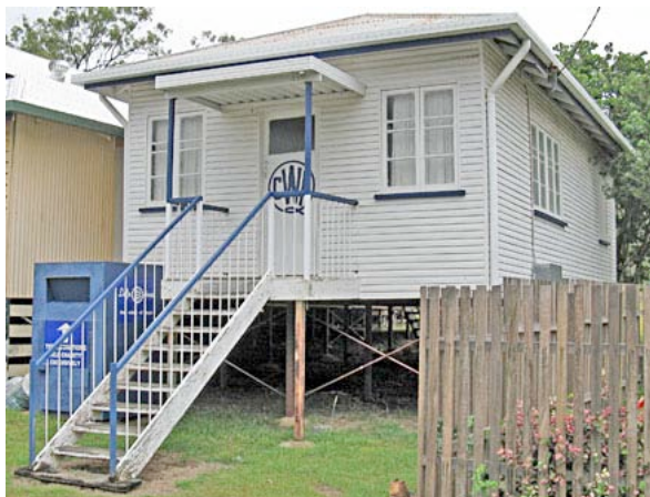
Front 3/4 views (above and below) showing small roof over entry, main hip roof, stumping and stairs. Originally the building likely had timber stumps and may have been closer to the ground.
