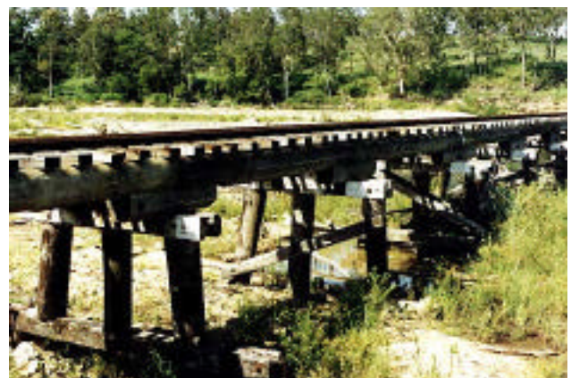
Cane line on ex-QR timber trestle (2 photos above).
