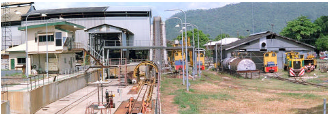
A mill in the early 1990s (above). Traffic officers in the elevated office (top left) schedule bin deliveries and oversee the weigh scale and rotary dump. Billets go up the conveyor belt to the crusher. The locomotive depot is top right.
