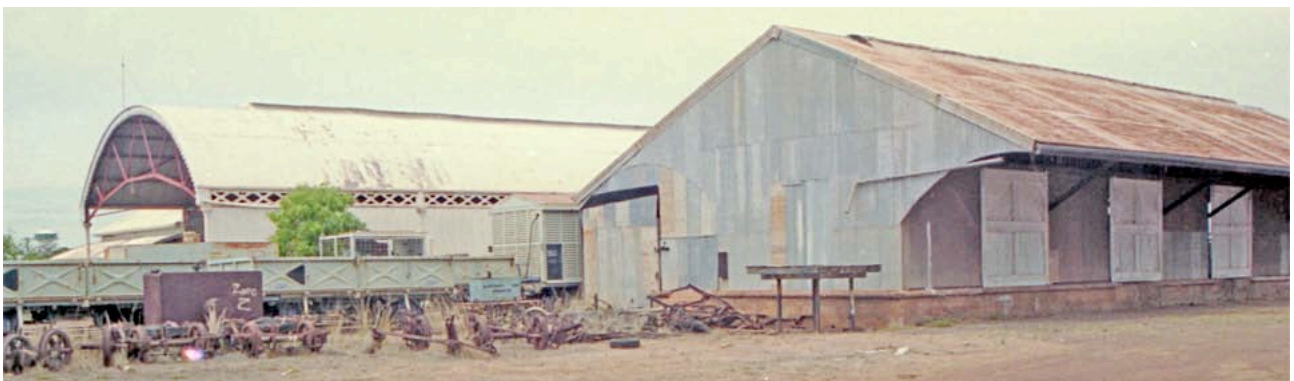
The large non-standard freight shed at Normanton, 1996. Jim Hutchinson, photographer.
