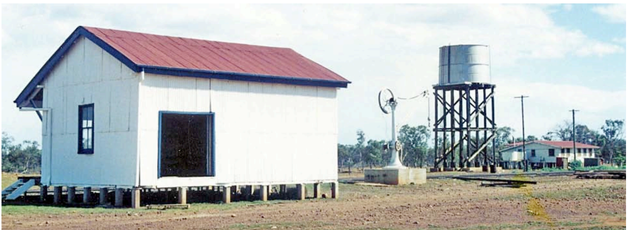
The yard at Cheepie with a standard 22' x 14' corrugated iron shed with a yard crane, 30,000 gallon water tank and barracks nearby, 1996. Jim Hutchinson, photographer.
