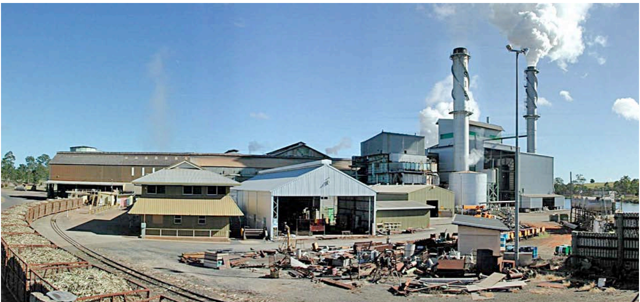
Isis Mill, August 2002. Loaded bins enter the weigh station and mill to left, passing in front of the traffic office.
