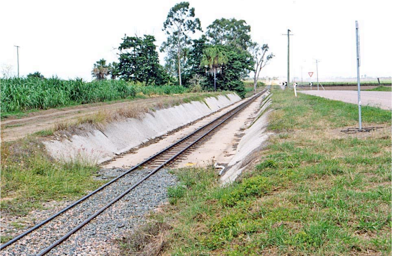
Cement lined cutting on the Kalamia Mill system
