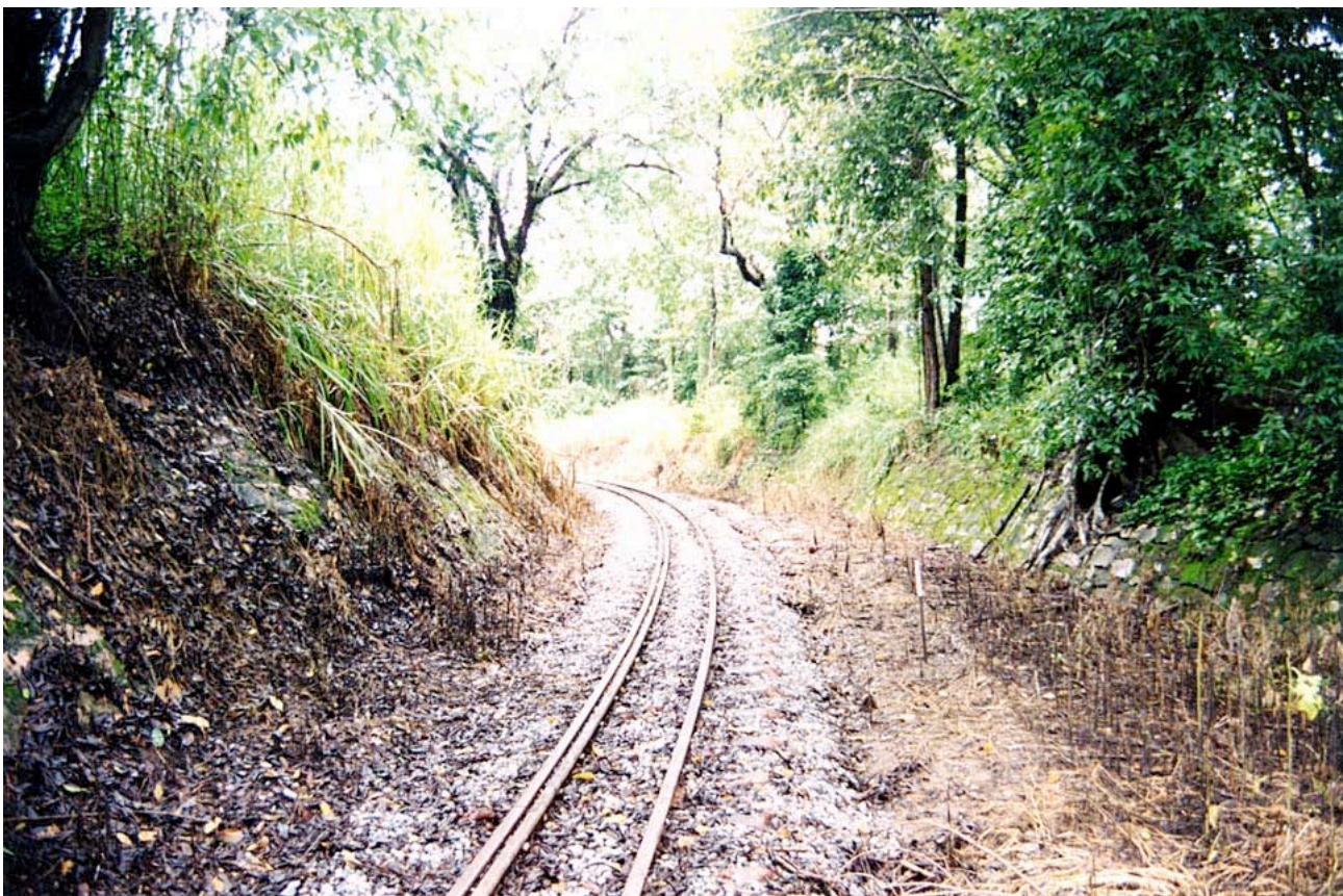
Cutting coming out of the Herbert River, Victoria Mill system
