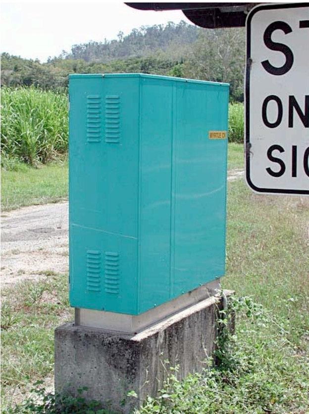
Active crossing control box near Proserpine; track sensors were also located some distance away on either side of the crossing. Signal lamps are often covered on less used lines during the off season. Lynn Zelmer, photographer
