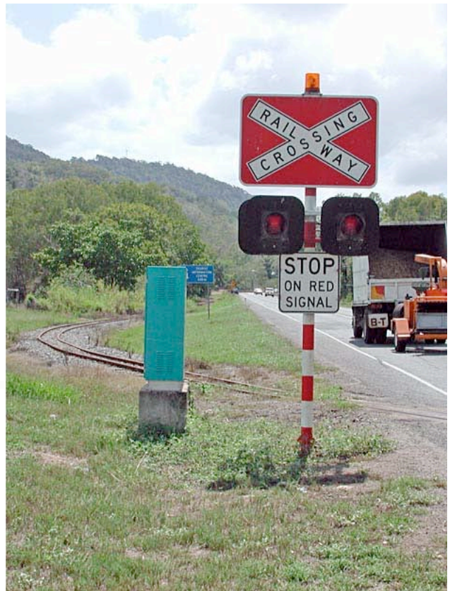
Active crossing control box near Proserpine; track sensors were also located some distance away on either side of the crossing. Signal lamps are often covered on less used lines during the off season. Lynn Zelmer, photographer
