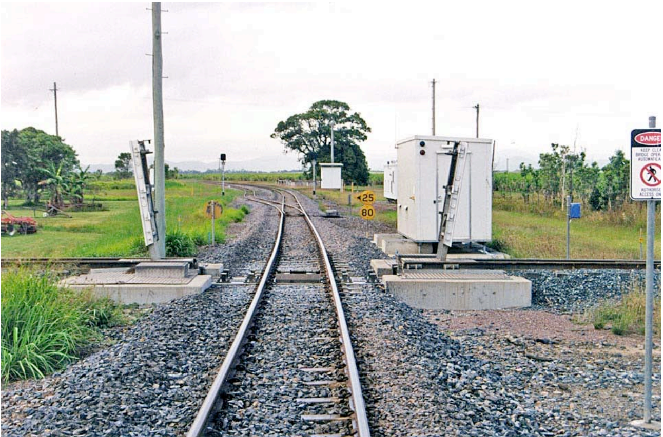
Drawbridge on the Racecourse mill system.
