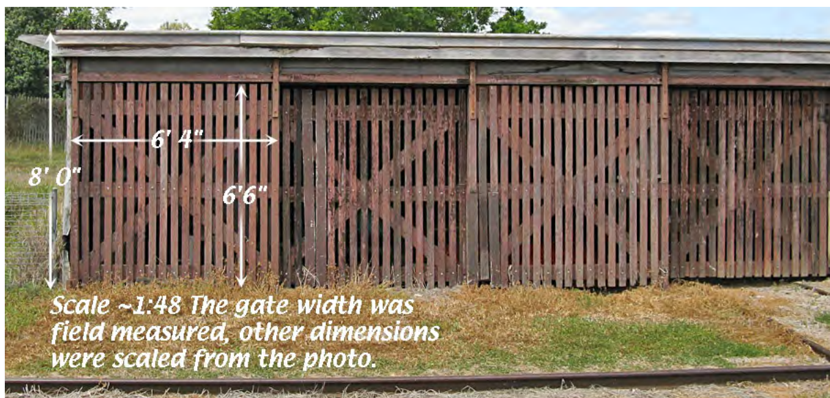
Basic dimensions for Mount Morgan fettler's shed.
