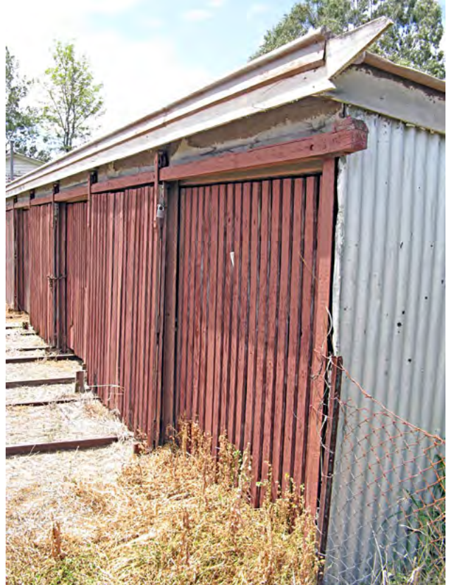
South end of the Mount Morgan fettler's shed, October 2008. Note the shape of the fascia board end and the painted sheathing. A door lock can be seen at the top of the first door, the lock on a door further along is at waist level..
