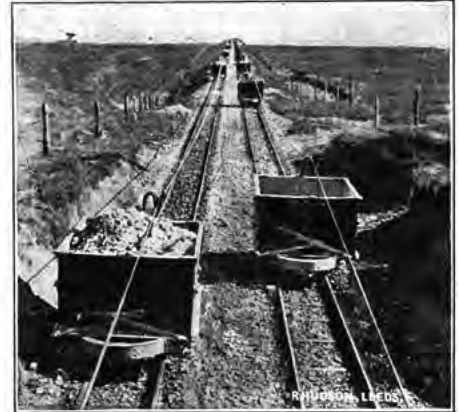
ENDLESS WIRE ROPE OVERHEAD hauling Hudson side discharge trucks by means of pivoted jockeys
