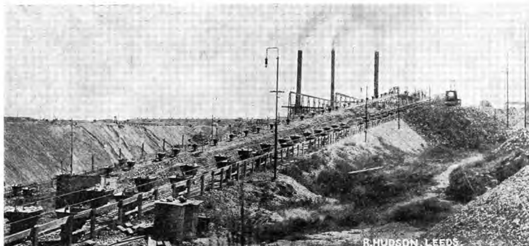
HUDSON SIDE TIPPING TRUCKS on main haulage of diamond mine
