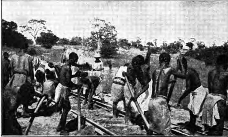
LAYING THE TRACK FOR THE LUANDA RAILWAY IN ANGOLA—P.W. AFRICA
