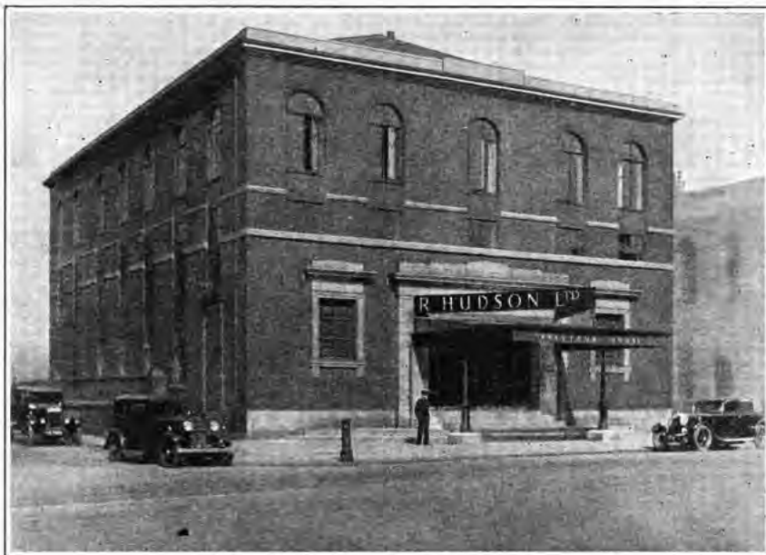
HEAD OFFICES OF ROBERT HUDSON LTD. "RALETRUX HOUSE," MEADOW LANE, LEEDS
