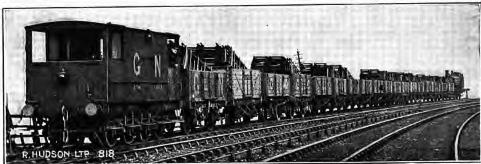
A 200 TON TRAIN LOAD OF HUDSON RIVETED TRACK LEAVING OUR WORKS SIDINGS AT GILDERSOME FOUNDRY
