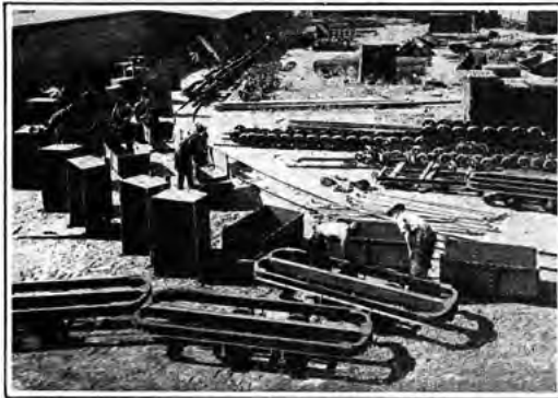
ERECTING HUDSON TRUCKS AT OUR DURBAN WORKS
