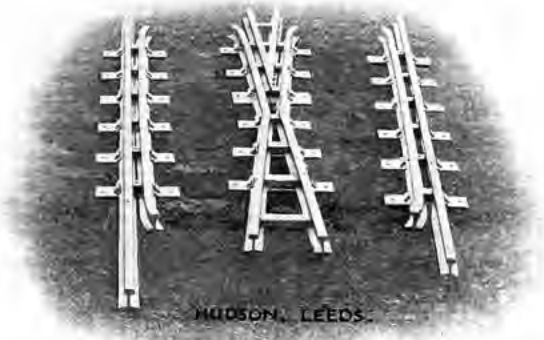
A FROG with two guard rails and two stock rails, etc.
