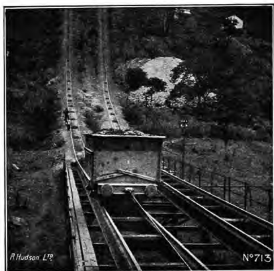
HUDSON SADDLE BACK HOPPER TRUCKS of 10 ton capacity descending a very steep grade on Rhodesian gold mine
