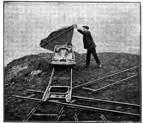
AS USED ON EMBANKMENTS—AVOIDING THE USE OF END-TIP WAGONS
