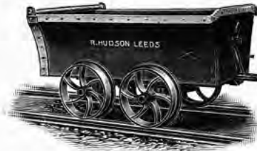
SMALL BOX TRUCK with end door, no buffers, through drawbar
