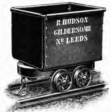
SMALL BOX TRUCK with end door, and buffers and couplings
