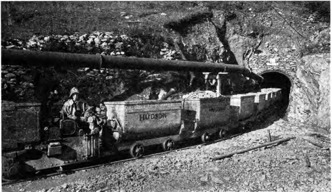
SIDE TIPPING WAGONS AT WORK ON A TUNNEL CONTRACT
