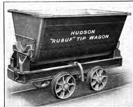
30 cu. ft. "V" shape, "RUBUF" type, body with flat top hoops Code 36471
