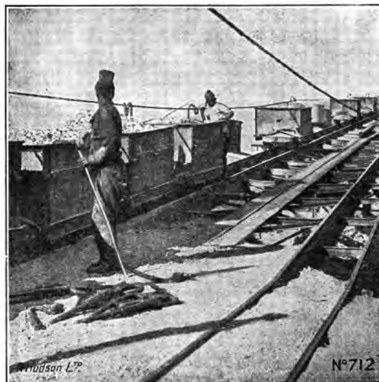
HUDSON SADDLE BACK HOPPER TRUCKS of 40 cubic feet capacity starting at foot of incline on African gold mine
