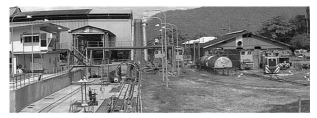
A mill in the early 1990s (above)... weigh scale and rotary dump (centre); billets go up the conveyor belt to the crusher; traffic officers in the elevated office (upper left) schedule bin deliveries. Locomotives are fuelled and serviced (right).
