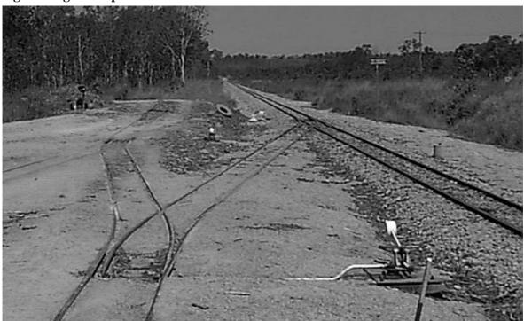
Contrast the well-maintained through line on the right with the pickup point and loop. The through line is at least as well engineered as the nearby QR mainline. The loading ramp is on the rise to the left of the old tire (upper left). Empty bins are left on the almost hidden line to the left, full bins roll down the center track. Note the wye point and the slight down grade to the through line.
