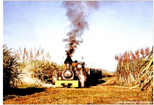
Most early trackwork was laid directly on the ground... without ballast or formation profile. Macknade Mill NQ, Hudswell Clarke 0-6-0 Seymour Line -- 8.69, John Browning Collection
