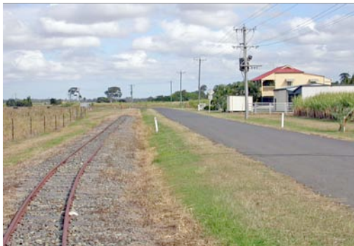
Bundaberg area, cane line running alongside the local road. Line is well maintained with reasonably fresh ballast and annual weed spraying. The line terminates in an unballasted and over-grown length of track before the road turns.
