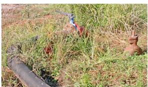
Permanent pipe with valve and connection to flexible pipe to pump. The valve and connection can be seen to the left of the pump in the photo above. Two steel posts identify the site for when the pump is not present.
