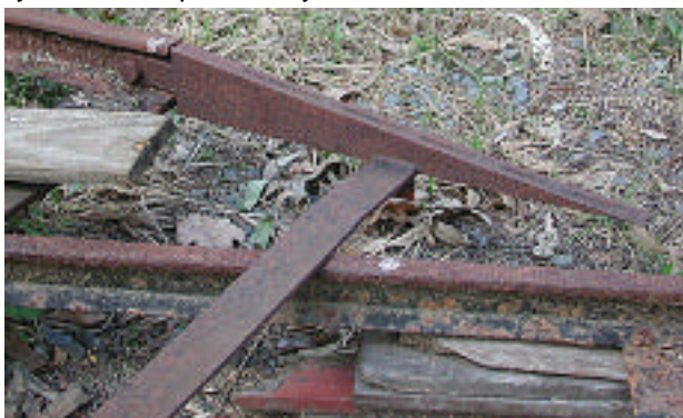
End of a curved 'climbing turnout', a special curved track to move between the permanent way and temporary tracks without requiring a regular turnout. This incline end was fitted over the permanent rails and bolted to the temporary field line so that a wagon/truck could be pushed up the incline and off into the cane field.
