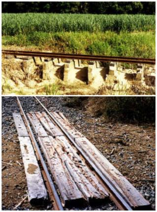
A rural grade crossing (above), the diagonal ruts through the timbers on the top crossing are the result of a derailment.
