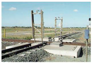
This drawbridge-type cane railway crossing of a high speed QR line near Mackay is remote controlled from Townsville. The cane tracks jog on both sides of the crossing and are fully protected by derails to prevent accidental movements. The bridge rails are roughly 2 m long.
