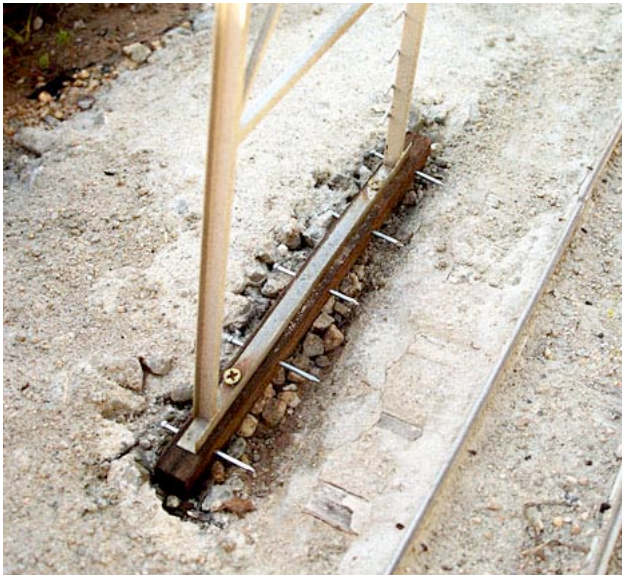
Foundation anchoring detail: the footer plate has two brass screws into 1/2 X 1/2 Redwood strips. The nails were installed to make a 'Rebar' to help anchor the footings. I drilled holes first, then inserted the nails so the wood wouldn't split.
