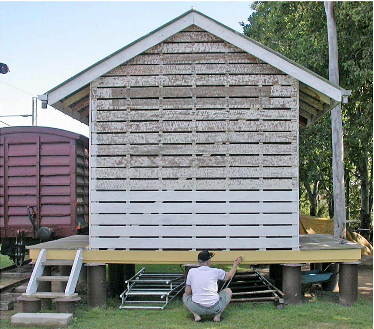
Note the location of the name board and the width of the diagonal brace, likely 1" x 3" timber inset into the vertical studs. While the exterior of the building (and outside edge of the studs, etc.) was painted white, the interior timber had either been painted a dark colour or had weathered dark. Lynn Zelmer photo, 2005.
