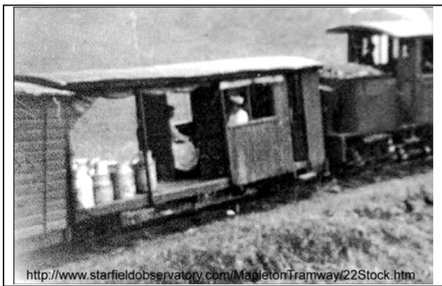
Shorter guard's van (left and below) with passenger accommodation and space for cream cans and other freight (left). The guard sorted mail into pigeon holes on the front bulkhead, and while there are foot steps on each side for the guard, there are none for the passengers. The van has a hand brake for the bogie under the guard's compartment. [Henworth]
