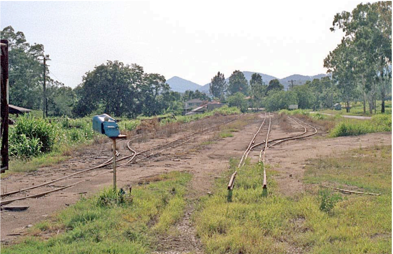
Truck/tractor dump on a lightly used line near Mackay. The blue box on the post is for bin tickets. Lynn Zelmer, photographer.
