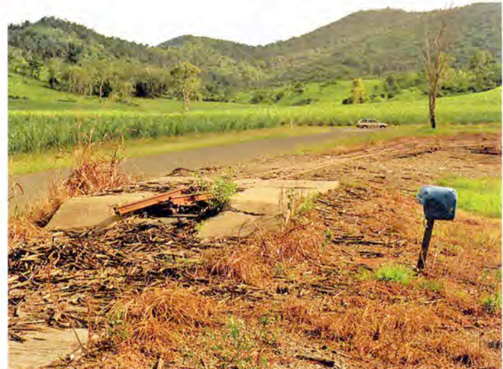
There is a single set of points dimly visible above the post, with another transfer point to the right so that gravity assists in loading the bins for the truck's return journey to where it can transfer the bins to the rail system. The cut-off plastic drum mounted on the post stores bin tickets for identifying the source and type of cane in the bin, delivery time, etc. Lynn Zelmer photographer.
