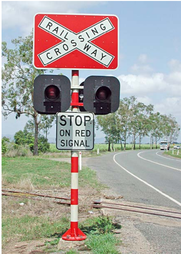
Standard cane railway level crossing lights: the oncoming train triggers the lights, which remain on until the train has crossed the road, Proserpine Mill, 2003. Lights at some crossings will also have an indicator light so that train crews can be assured that the lights are working.
