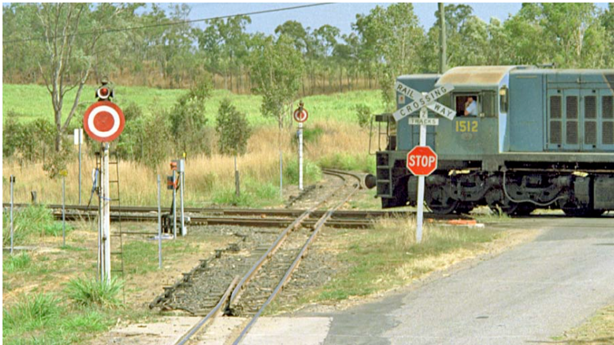
Mackay Sugar level crossing QR's North Coast line, 1998. The combined stop and railway sign is obviously for the shire road; the target and lights protect QR from the cane railway. Clearance must be obtained required from the QR controller, before the derails can be reset to allow the cane train to proceed.
