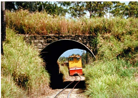
Underpass for a shire road near Finch Hatton, 1986. Greg Stephenson, photographer
