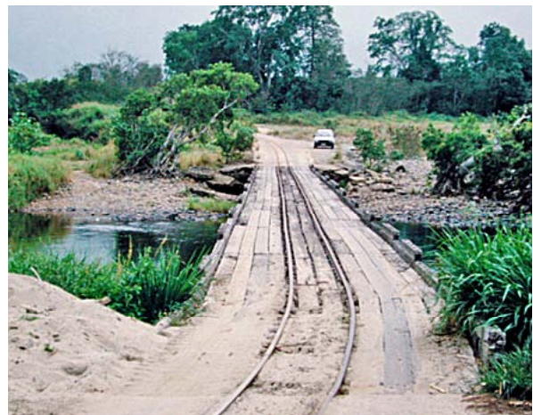
There likely are 'Yield' signs where the cane track joins the shire road but neither bridge nor tram line is marked on the approach to this shared road/rail bridge, likely Mulgrave Mill area c 1990. Greg Stephenson, photographer.
