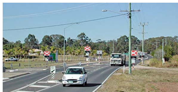
Signs and flashing lights protect cane railway level crossing with semi-rural road. Near Bli Bli, 2002.
