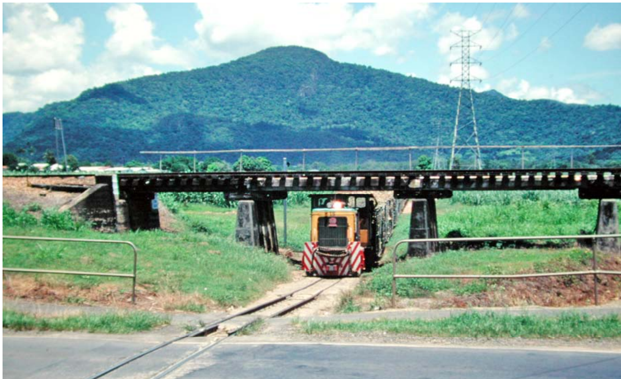
Mulgrave Mill grade separation with QR, Redlynch; 1995. Locomotives used on this line require reduced height cabs to allow them to pass under the QR formation. Greg Stephenson, photographer.
