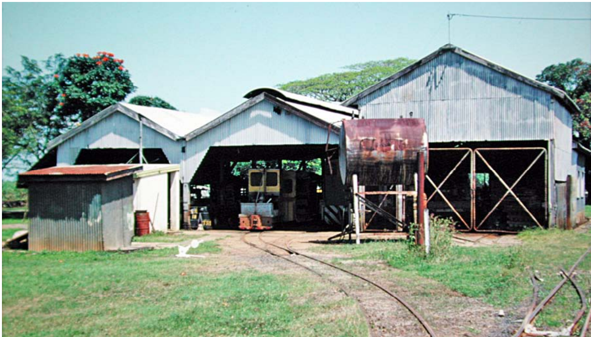
Goondi Mill loco shed being used as an out-depot of Mourilyan Mill, 3 October 1994. This complex was severely damaged by Cyclone Larry in March 2006 and was subsequently demolished. Greg Stephenson, photographer from the CaneSIG web site.
