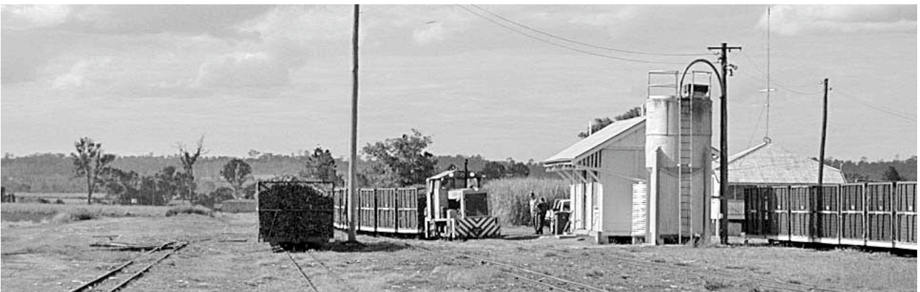
Bingera Mill's Sharon (ComEng 0-6-0 DH of 1959) at the Wallaville out-depot, located on the ex-QR formation, 2003. The ex-QR station, sand dryer, diesel bowser and storage tank (far side of building) and nearby fenced loco compound makes up the out-depot. Empty bins are despatched from here to the several out-lying branches and full rakes of cane are assembled for heavier locos to transfer over a grade to the mill. Lynn Zelmer, photographer.
