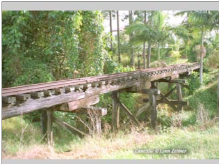
This is an ex-government railway bridge, with the cane railway running on the now-closed standard gauge (3' 6") railway formation.
