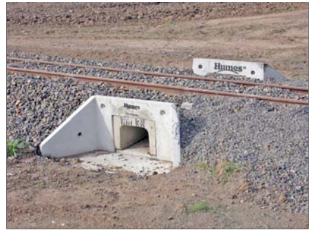
Precast drains and culverts make new construction easy c 2006.
