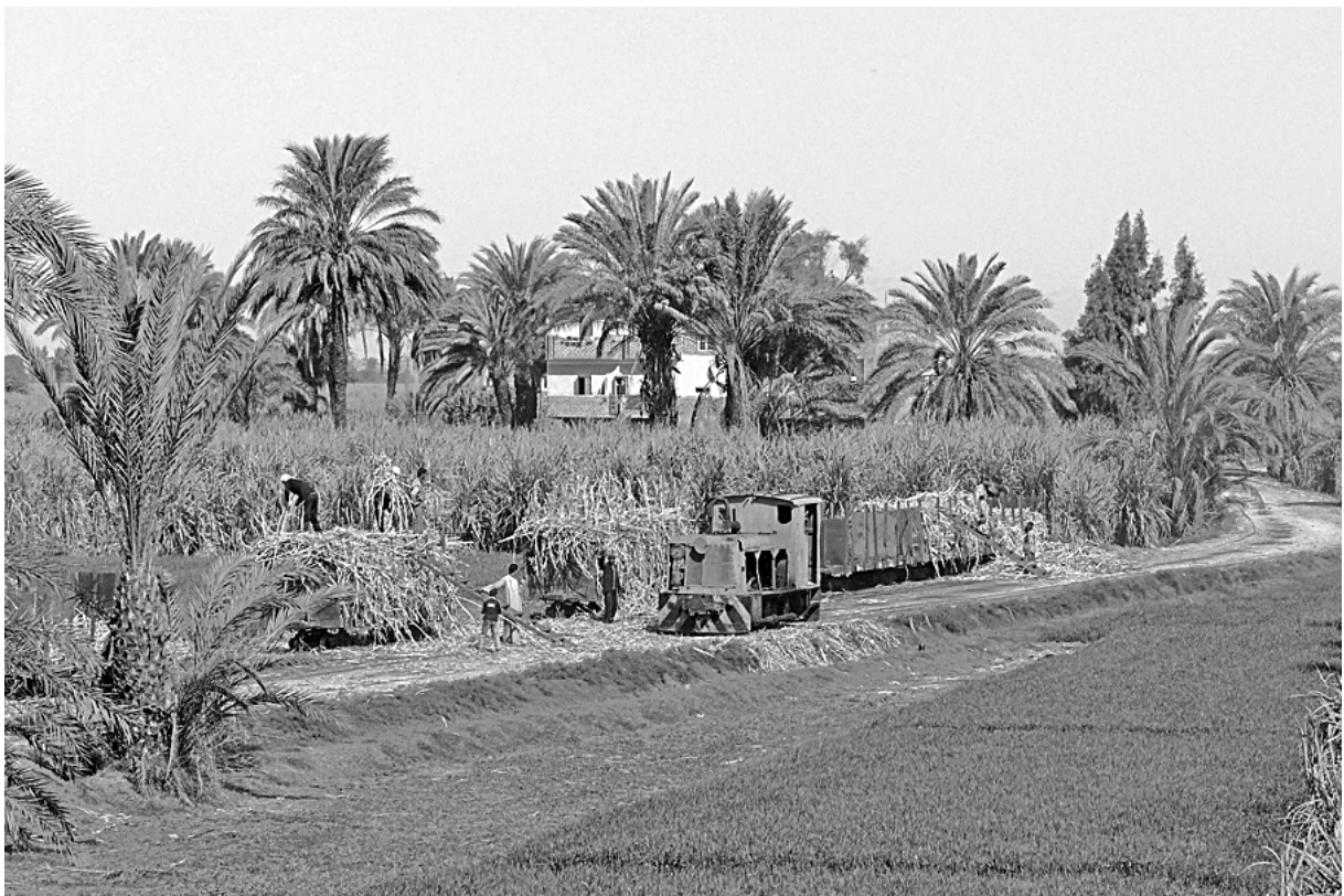
Egypt: Dishna Sugar Factory, #1 JENBACHER (Austria). Martin Heier photographer, 2009.
