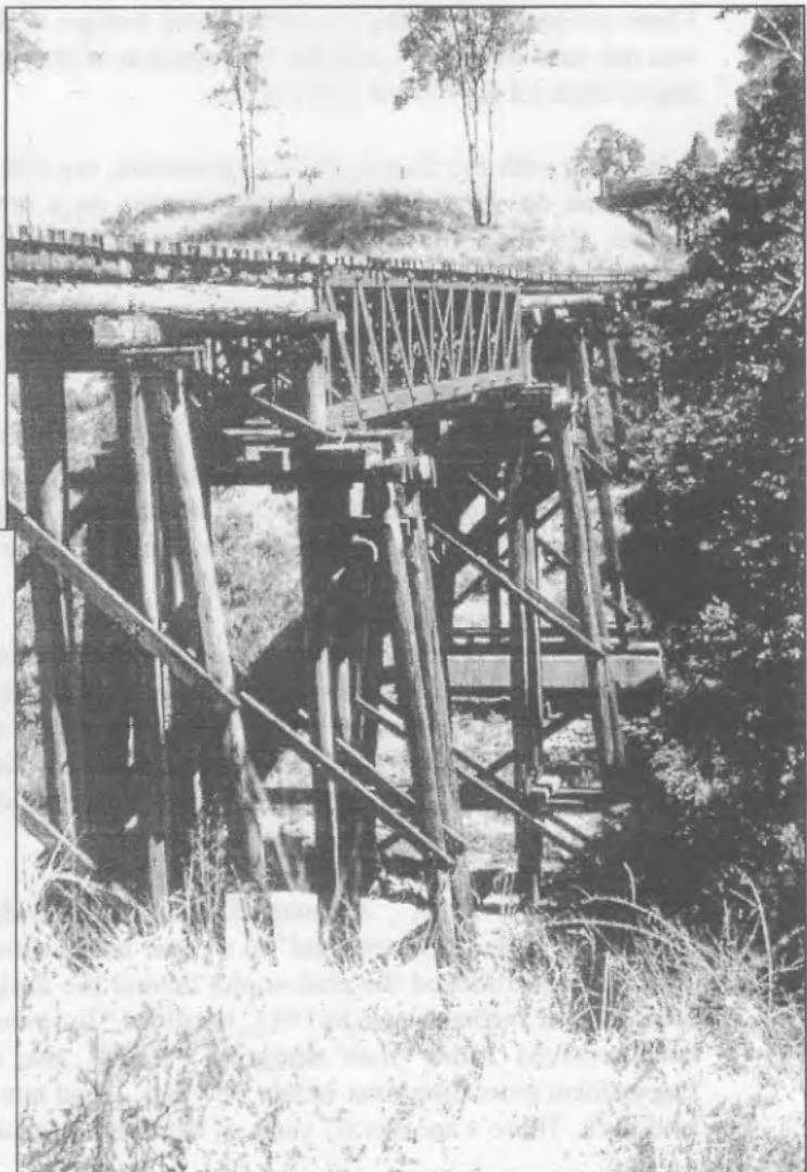
QR Bridge at Yandina. An example of timber approach spans to the steel main span. Also illustrated are repairs of ground line rot of the piles by installation of concrete sills at ground level on some of the piers. The timber spans consist of double girders.
