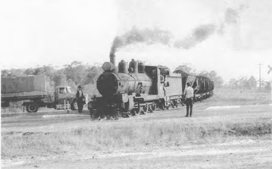
PB15 No 455 brings a load of coal into Dinmore, crossing the Brisbane-Ipswich highway just prior to entering Dinmore yard. The flagman to the left of the engine stopped road traffic while the train moved slowly across.
