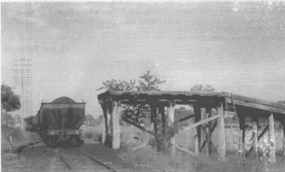
One of three coal loading rams at Walloon - two on the up side of the main line and one on the down side. Motor trucks reversed up the ramp and tipped coal into the hoppers placed adjacent to the ramp. Empty hoppers were positioned and full hoppers moved on by hand using a pinch bar under the wheels of the wagons.
