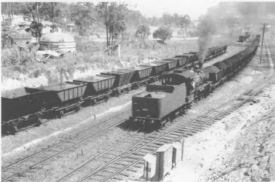
Running tender first, B18½ No 889 moves a load of coal on the main line through Dinmore. The empty hoppers to the left are waiting to be taken by one of the shunt trains to New Whitwood Colliery for loading.
