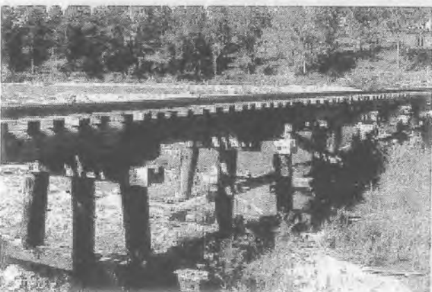
Cane line on ex-QR timber trestle (2 photos above) and on a cane railway-built bridge (below).
