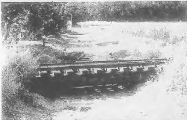
Low spot filled in with de-barked logs but no sleepers (above) and a proper dressed timber crossing with sleepers (below).
