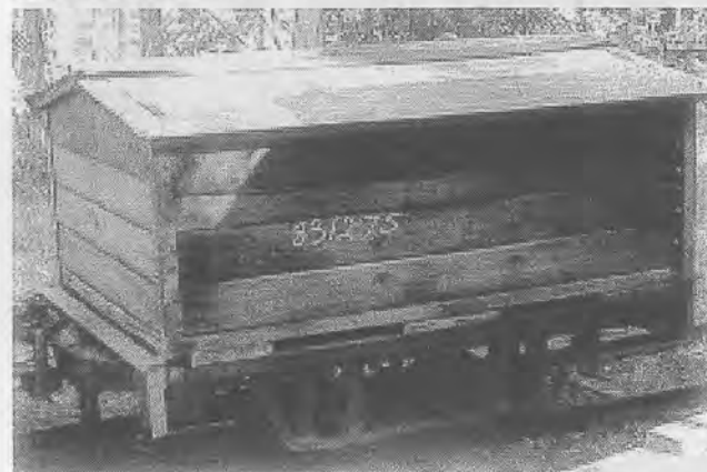
Wooden tool box on a wholestick cane truck chassis (ILLRS).
