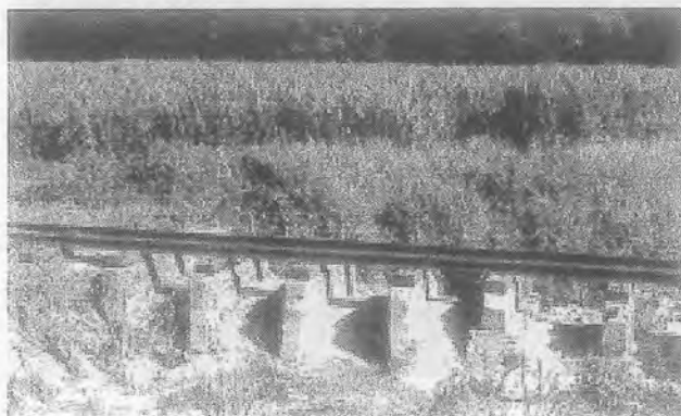
Steel girder on concrete risers (above and below); the gauge is maintained with welded braces, rather than sleepers. This was the inspiration for the small bridge on one of the ANGRMS dioramas.
