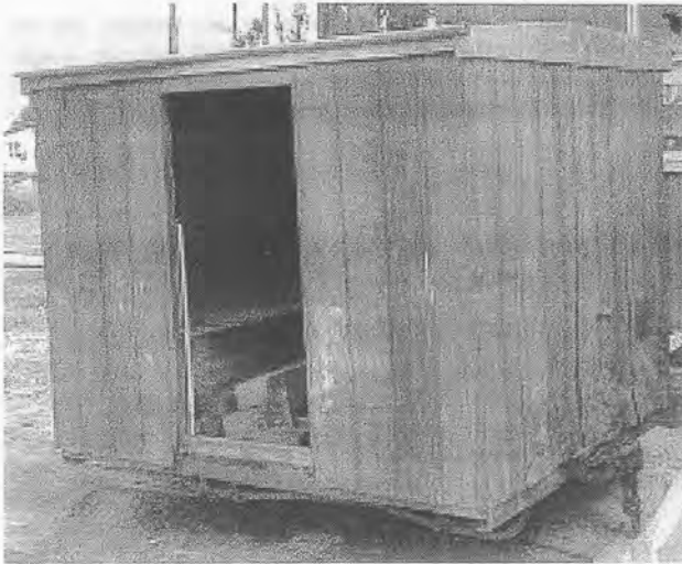
Aluminium sheathed tool shed on a cane bin chassis. The white object propped against the door frame is a metre stick.
