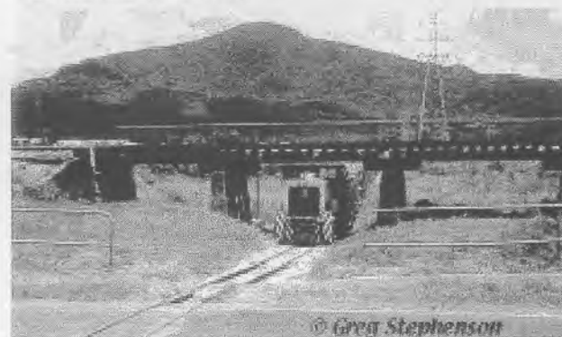
The cane railway underpass (above) eliminates the crossing but requires a lowered roof on locomotive cabs.
