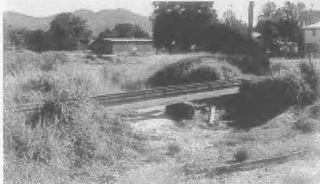
Steel girder on concrete risers (above and below); the gauge is maintained with welded braces, rather than sleepers. This was the inspiration for the small bridge on one of the ANGRMS dioramas.
