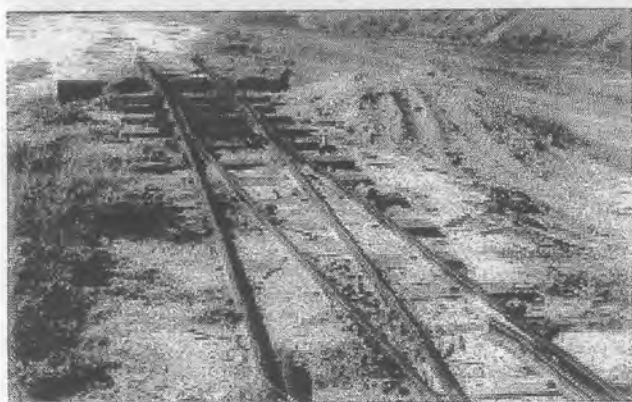
A concrete transfer ramp (above) and two views of a simple timber transfer ramp (below). A tractor pulls a trailer with bins over the ramp above, and parallel to the track below (wheel marks in the dirt pile), then backs into place. A guide pan on the back of the trailer lifts the hinged rail section into place.
