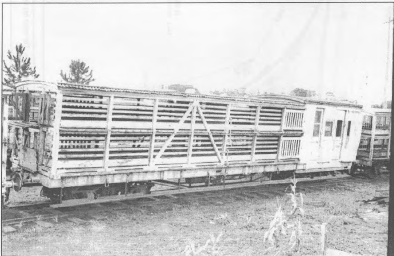
The NWB sheep wagon had the drovers and guards compartments at one end to allow continuous end loading.
