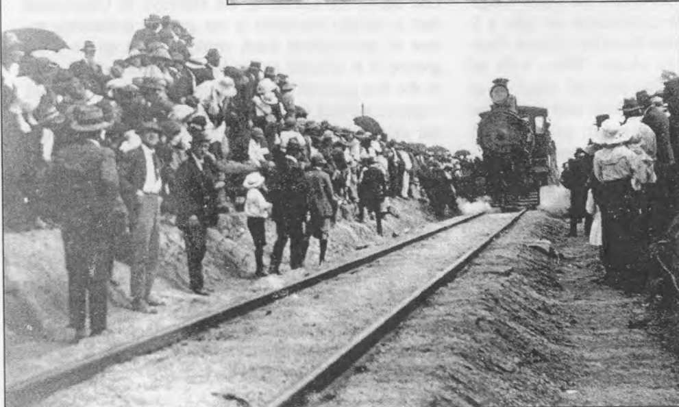
A good example of standard track construction in the early 1900's. Once again note the staggered rail joints. Photo: Courtesy John Oxely Library.
