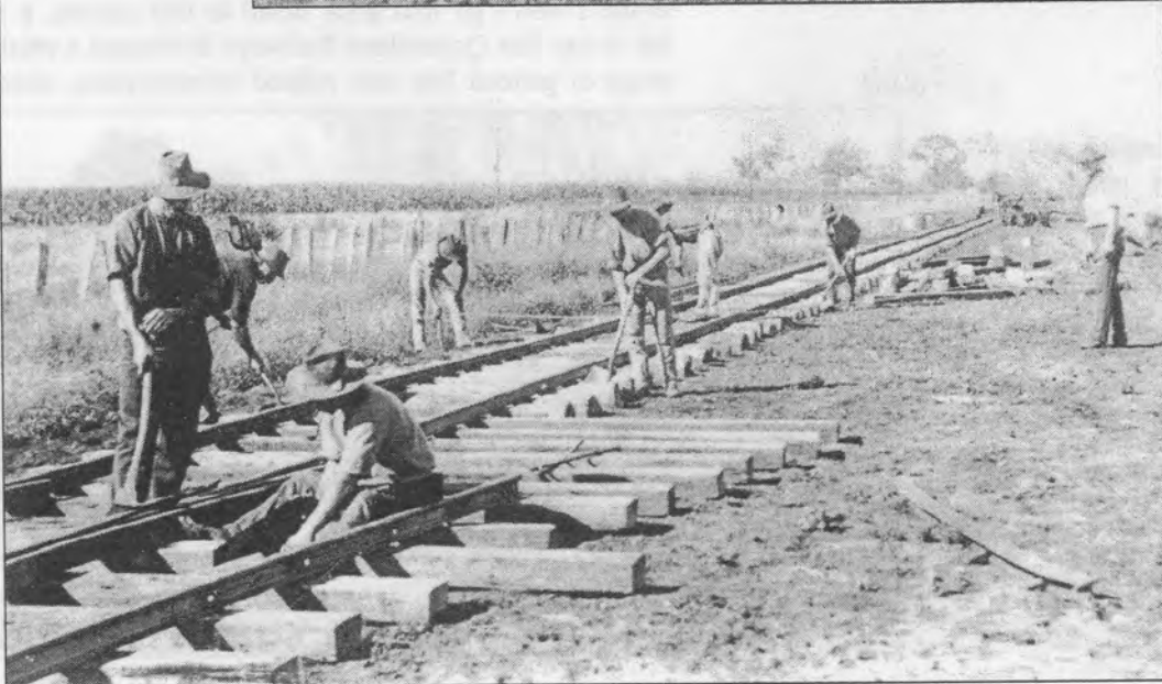
Construction of pointwork underway on the Pittsworth to Millmerran branch line. Photo: Courtesy John Oxley Library.
