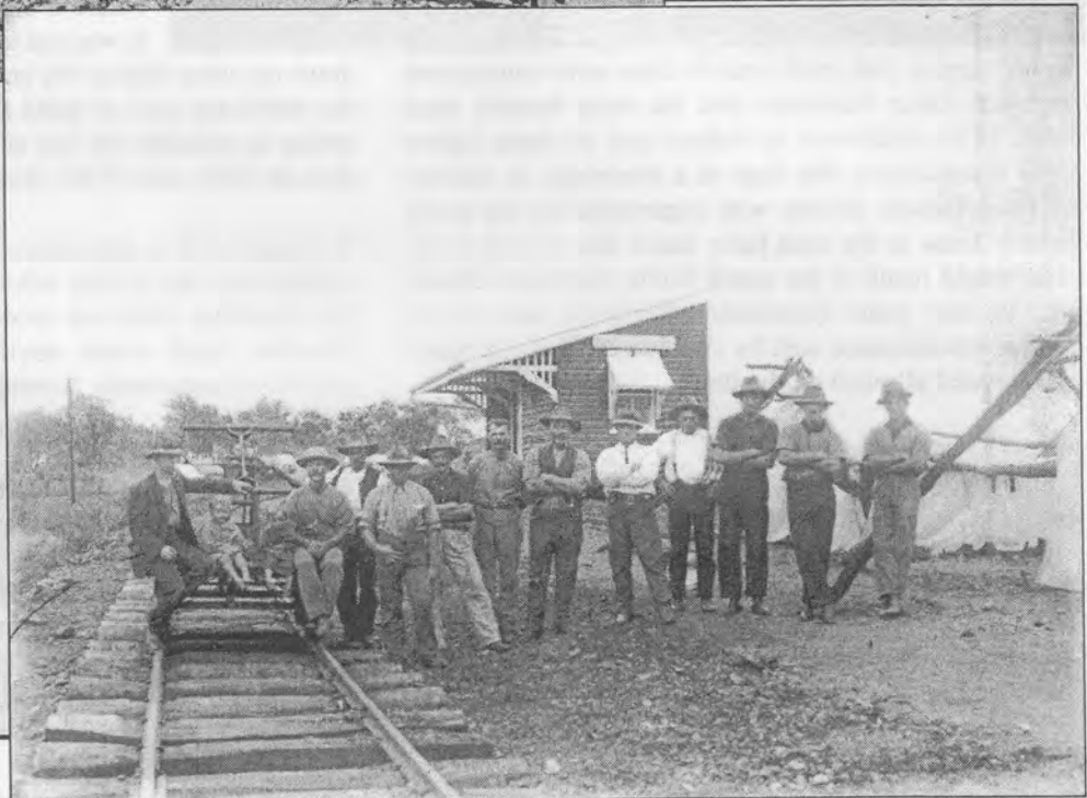
Freshly laid track on the Pitts- worth to Millmerran branch line. Note the rounded sleep- ers adzed to accept the 42 lb rail. The trackwork is yet to be ballasted. You can also see that the joints for the rails are staggered. Photo: Courtesy John Oxely Library.
