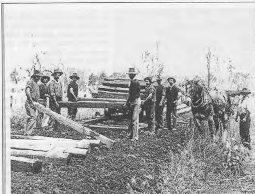
A track construction gang laying standard hardwood sleepers onto an already prepared road bed.
