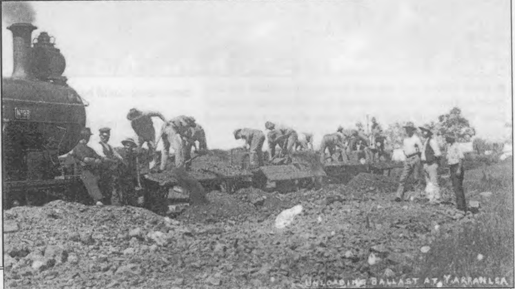
A ballast train being unloaded on the Pittsworth to Millmerran branchline. Note the irregular nature of the ballast, clearly not blue metal or crushed rock. Photo: Courtesy John Oxley Library.
