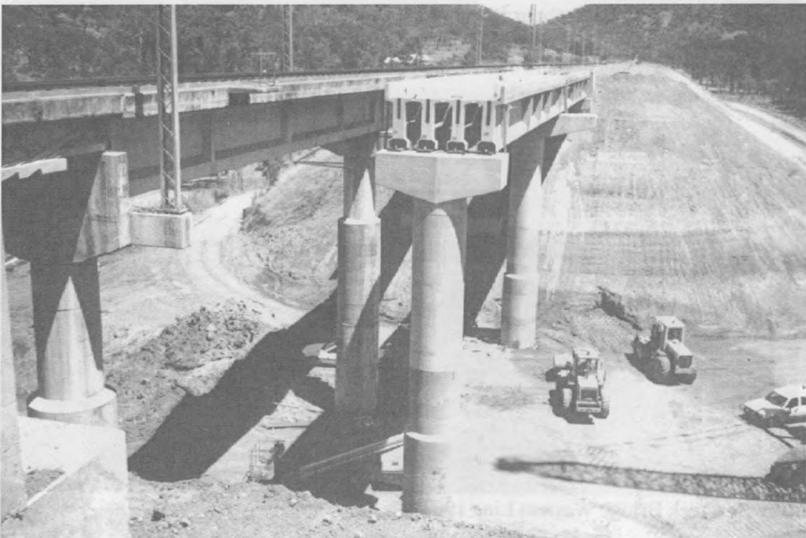
1997 prestressed concrete bridge of three 25m spans. Note the increase in pier diameter at the base on the high piers.
