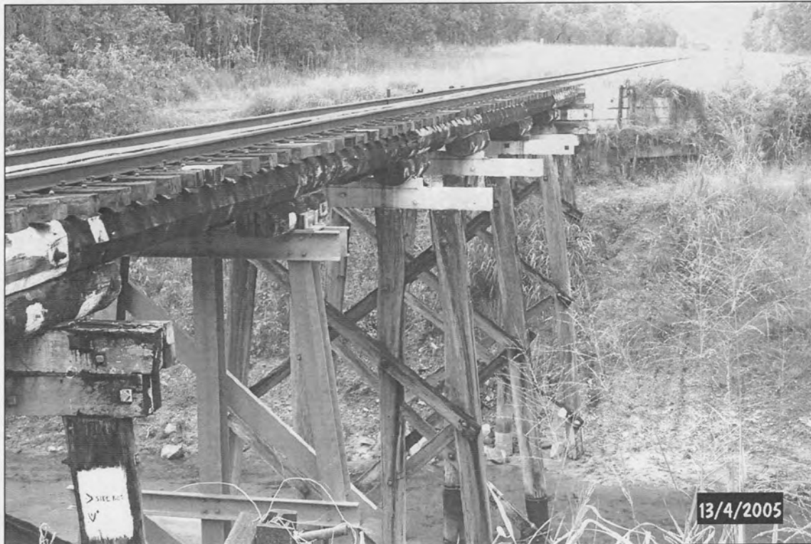
Replacement pier in steel.
