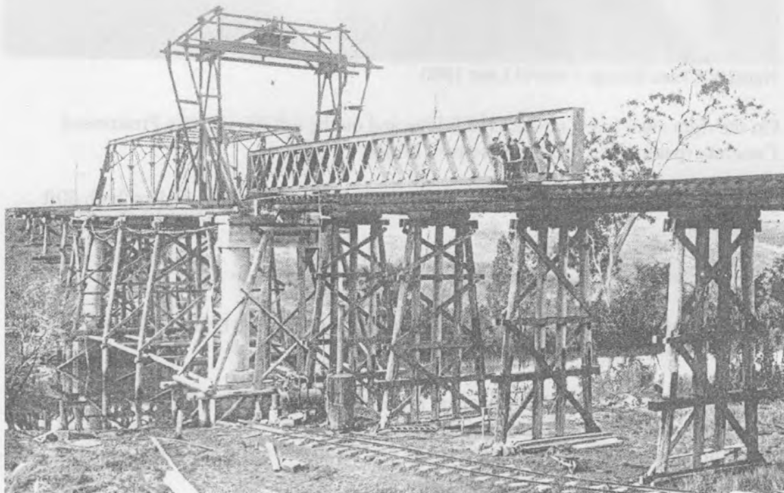
Grahams Creek Bridge North Coast Line ca 1916, removing original truss
