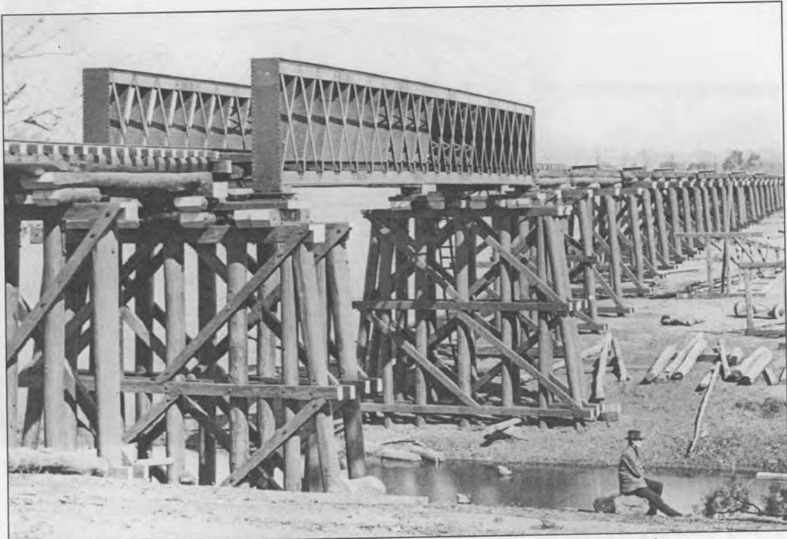
Condamine River Warwick 100ft (30.5m) span Lattice Truss on timber piers.
