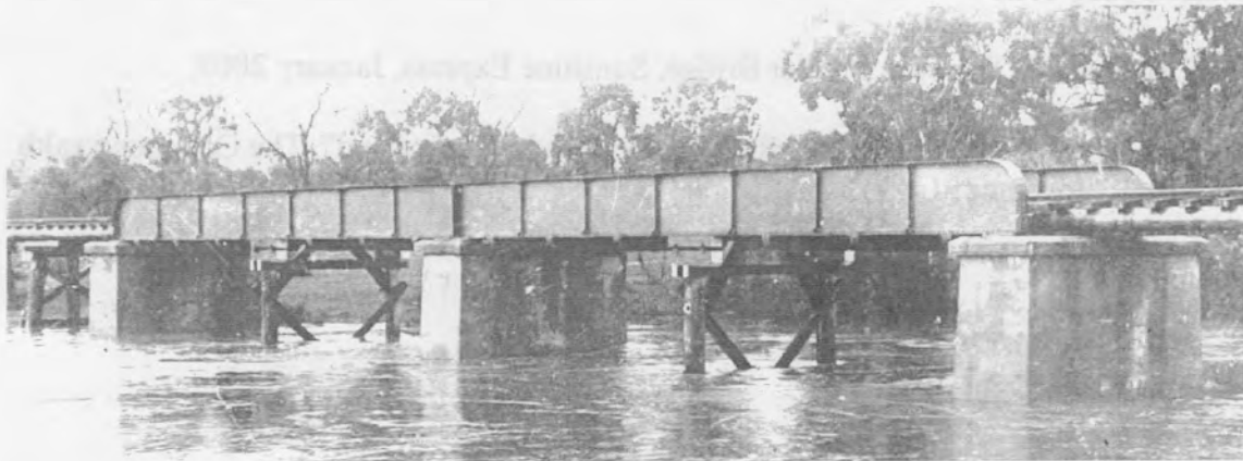
Accommodation Creek Bridge Southern Line 1902 Temporary timber piers pending the construction of the new bridge.
