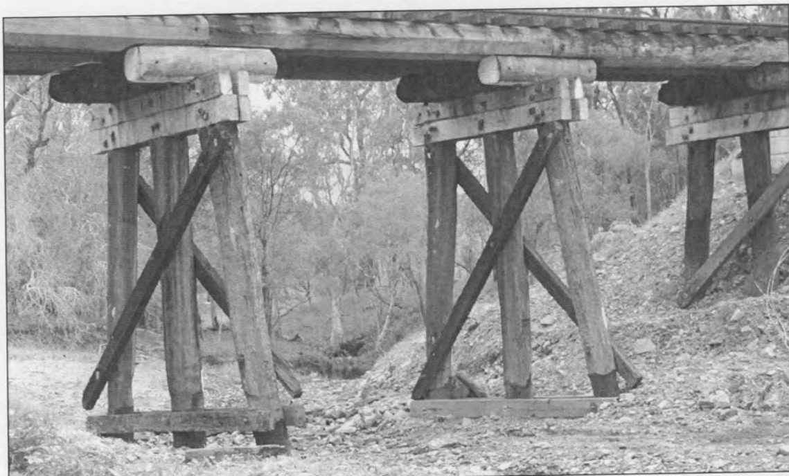
Double Headstocks on Timber Bridge
