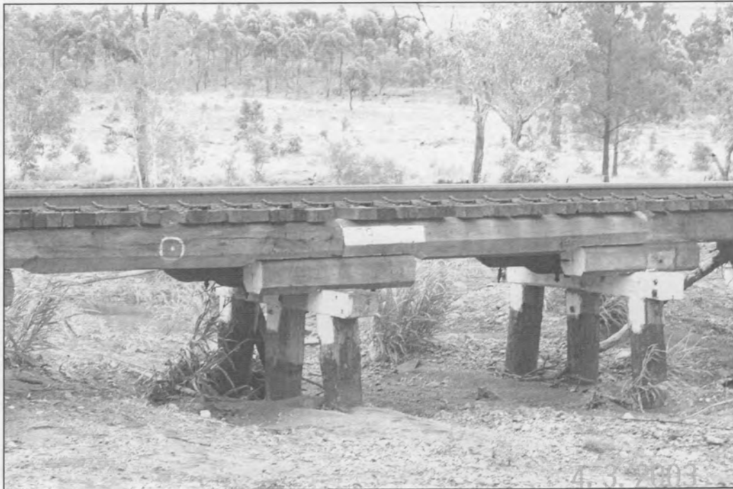
A timber bridge with solid headstocks ca 2000.
