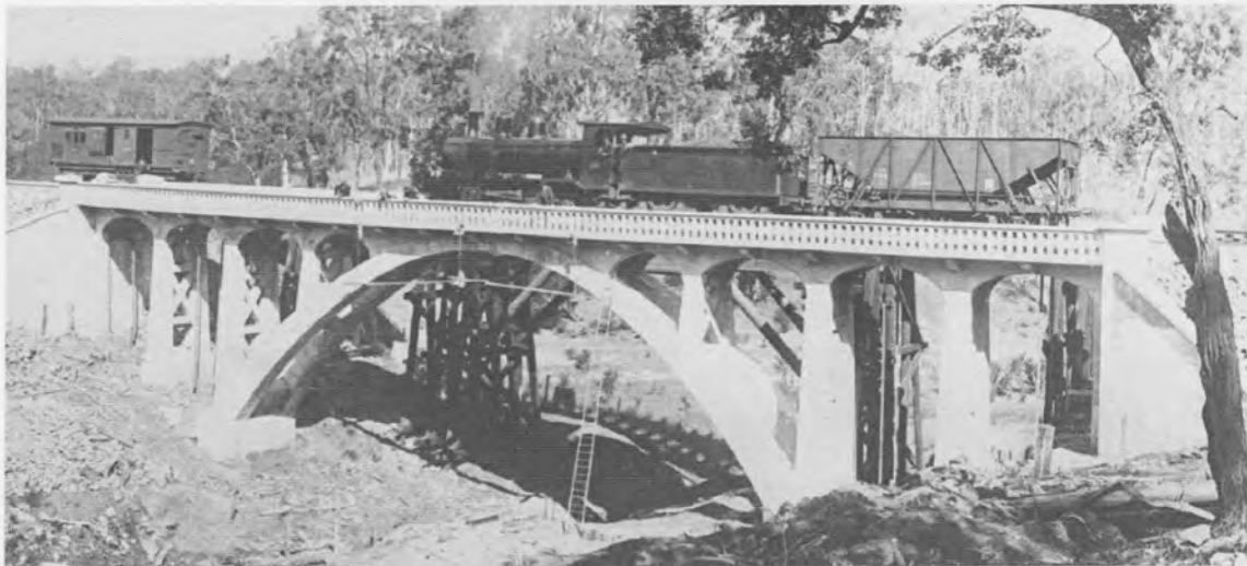
Concrete Arch Bridge at 75M 25c Main Line 1902.
