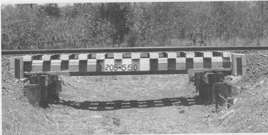
Again on the Western Line this is a simple single span bridge with concrete ballast boards.
