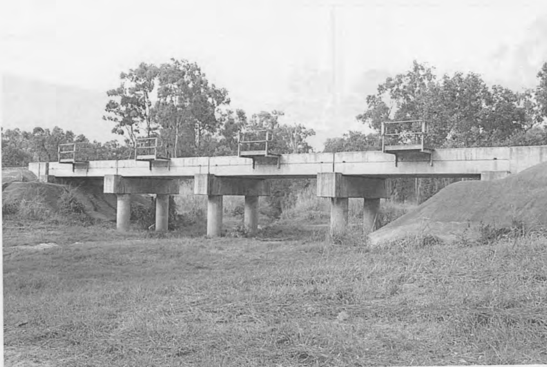
Prestressed Concrete Box Girder 1362.12km North Coast Line
