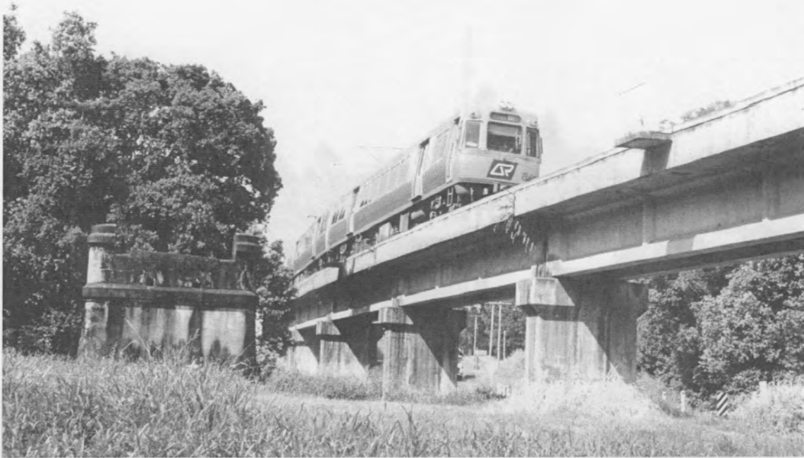
1966 prestressed concrete bridge of seven 50ft (15.2) spans on a curve. Concrete pier of old steel span on the left of the photo.
