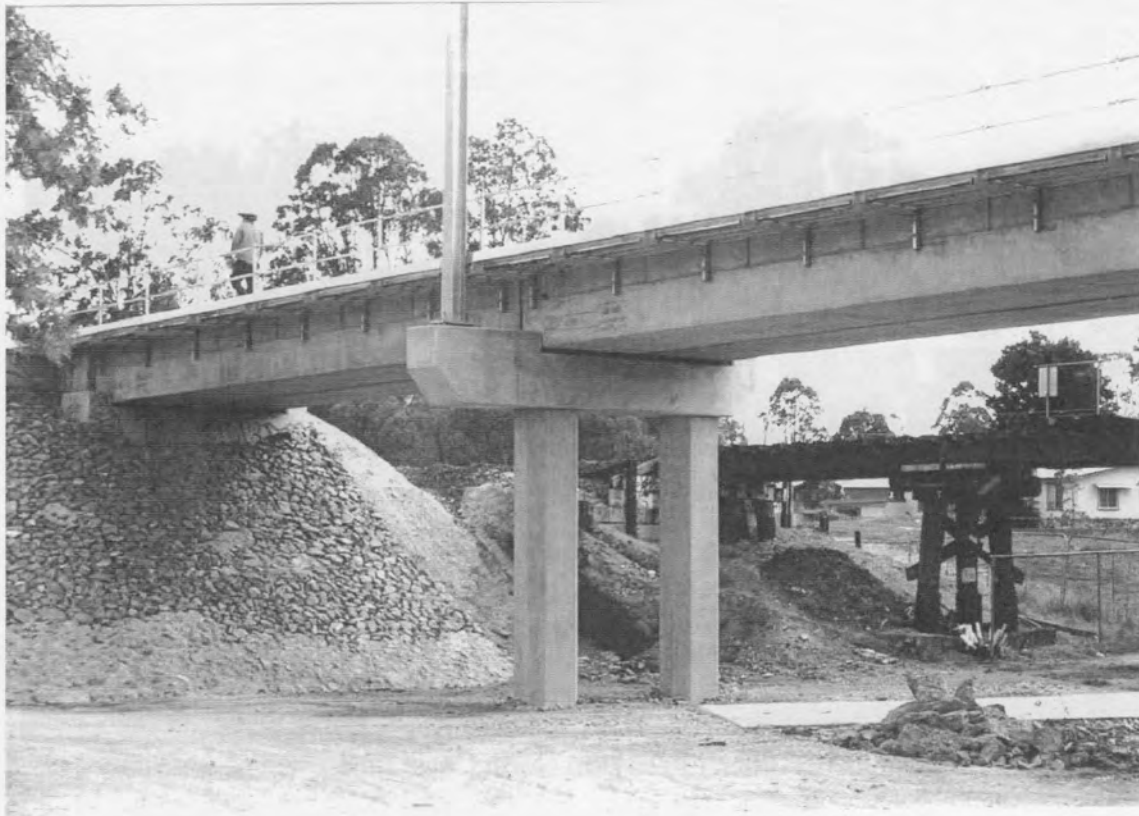
Hindes Street Bridge Lota 2007. Twin rectangular columns to piers.
