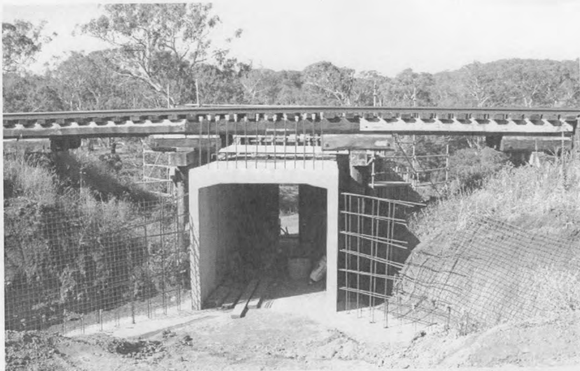
Timber bridge replacement by concrete culvert. In this case a large box culvert to provide access under the track.
