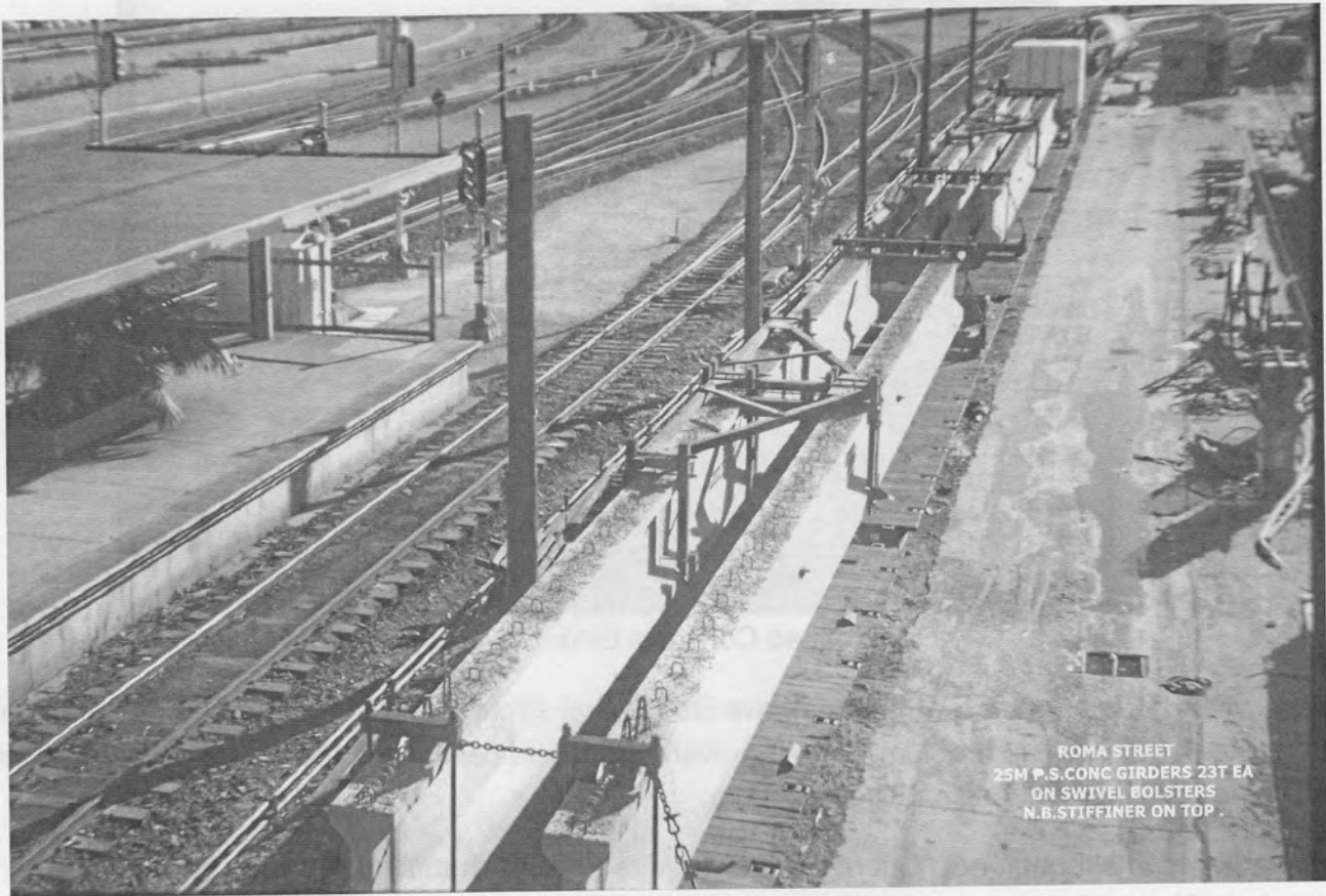
25 Metre P.S. Concrete Girders
