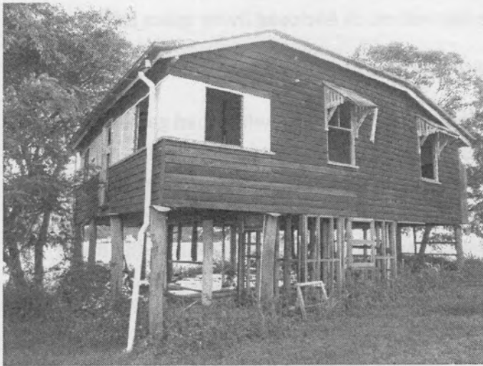
CAPALABA; LINSEED OIL WAS APPLIED TO THE EXTERIOR, NOT PAINT.
