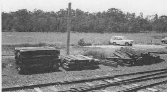
Stacks of sleepers along the line-how do they get there? Goods train with FJS loads stops and unloads them.
