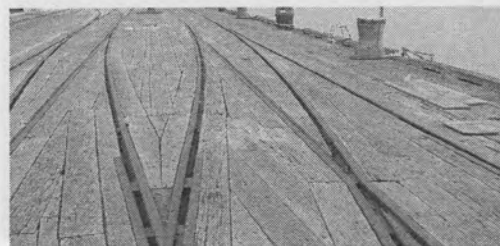
Typical dock setting of rails inside wood decking
