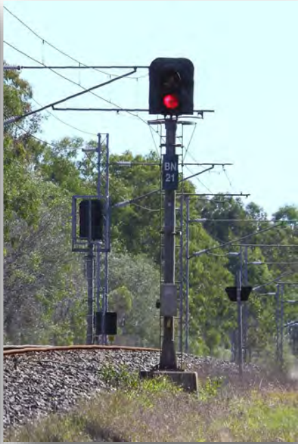
Down Advance Starter Signal
