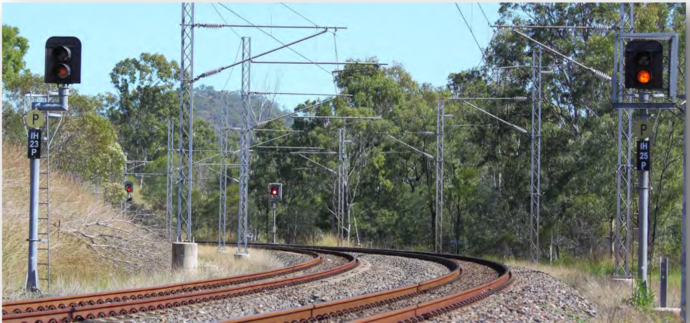
Loop and Mainline Repeat Signals (Repeating Starting Signals due to reduced sighting distance)
