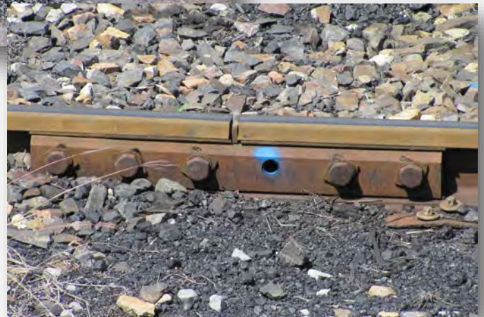
Insulated Rail Joint (Mechanical)
