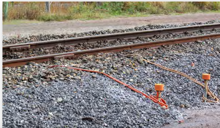
Insulated Rail Joints, Track Circuit leads & Track Connection Boxes
