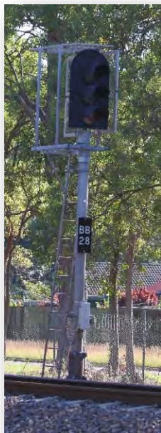
Down Outer Home Signal
