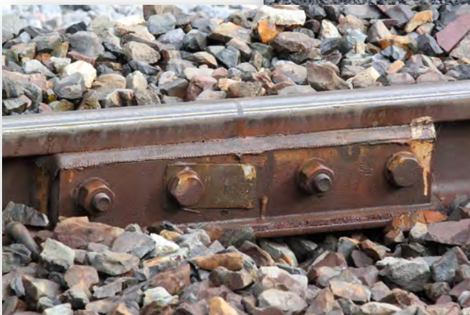
Insulated Rail Joint (Glued)
