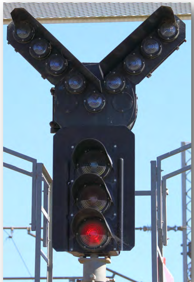
3 Aspect Signal with Multiple JRI (Position 1 & 4)
