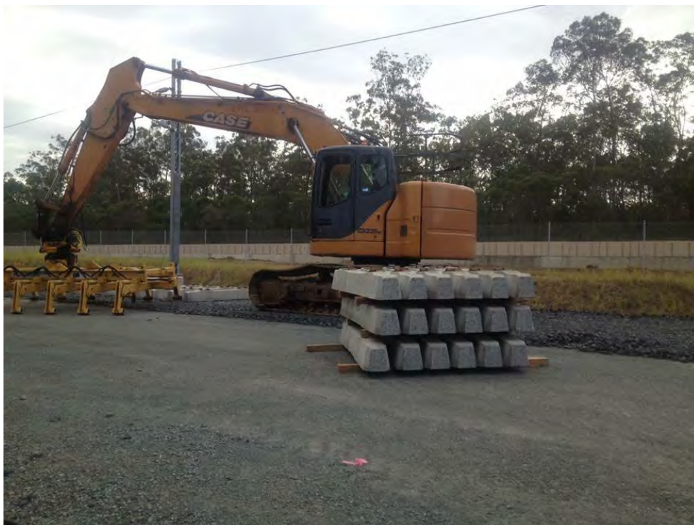
Concrete sleepers being placed on prepared trackbed.
