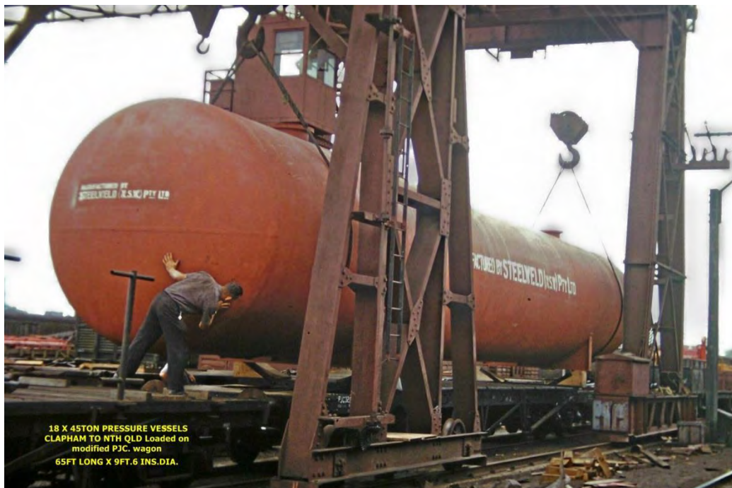
The Gantry at Clapham was used for loading this 45 Ton Pressure Vessel onto a modified PJC wagon.
