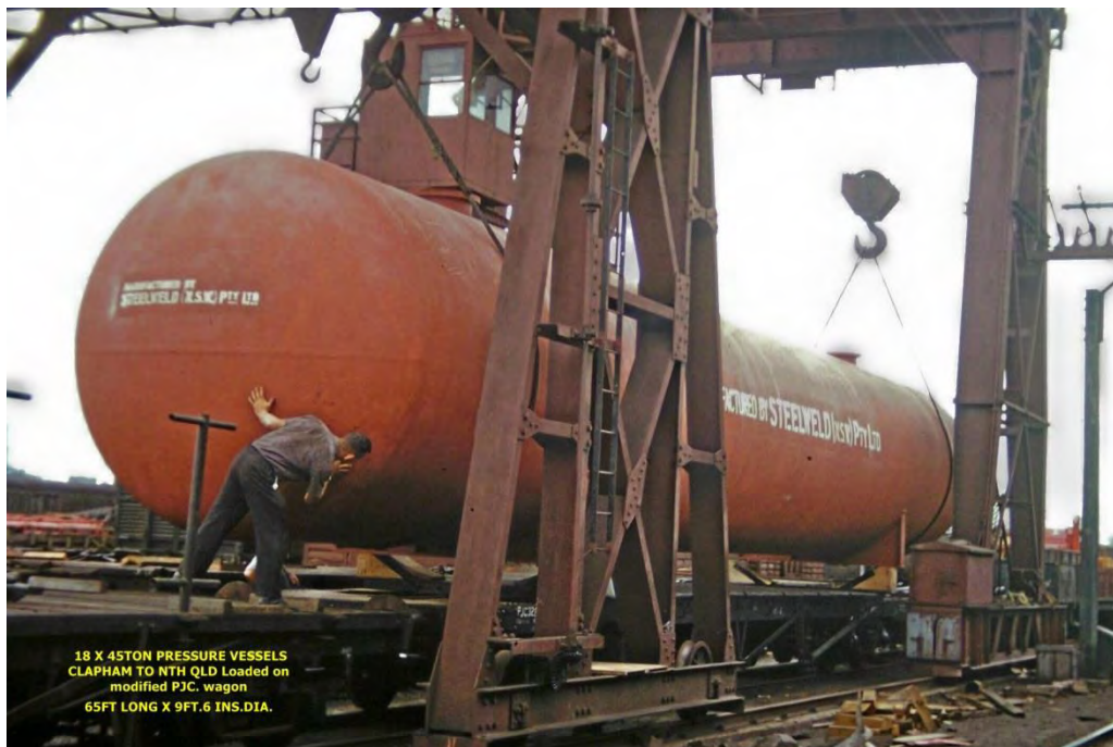
An overhead Gantry being used to load a 65 foot long Pressure Vessel for North Queensland onto a modified PJC wagon at Clapham.
