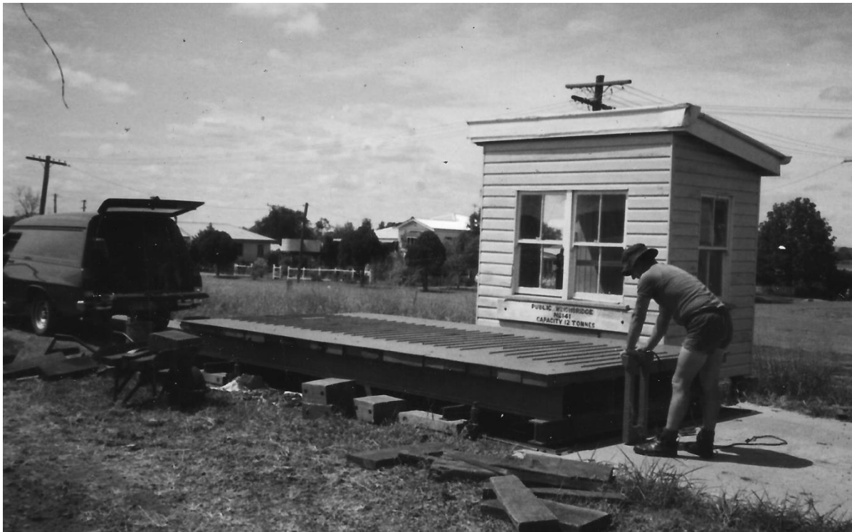
Thangool Weighbridge being serviced on 21 st February 1983e
