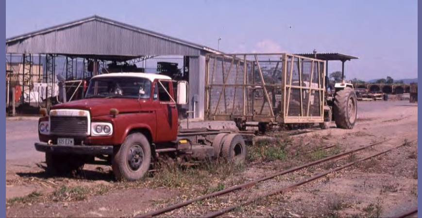
Transfer from truck to tramway
