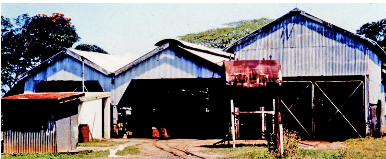
The former Goondi 'triple-fronted' steam shed serves as an out-depot of Mourilyan Mill. The central bay accommodates the two-road loco shed, with the left and right hand bays housing workshop, storage and navvy facilities. Greg Stephenson photo, 1995.
