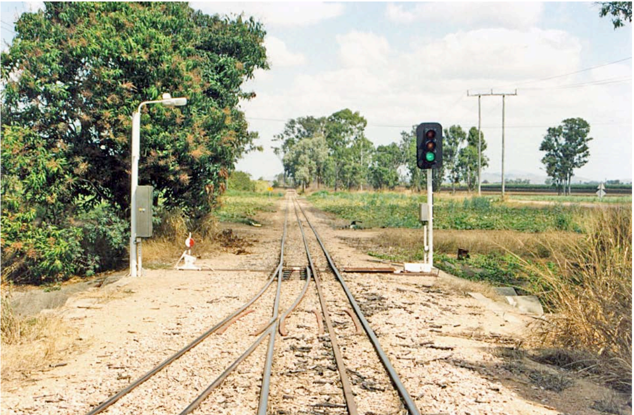
Automatic points at Airdale where the Kalamia and Pioneer systems combine.
