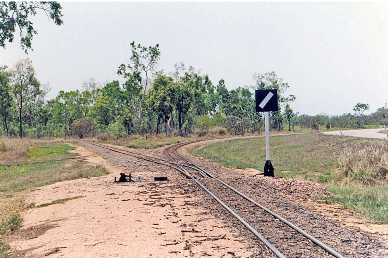
Point indicator on the Invicta Mill system at McLain Road Junction. The same type of indicator is used for trailable points.
