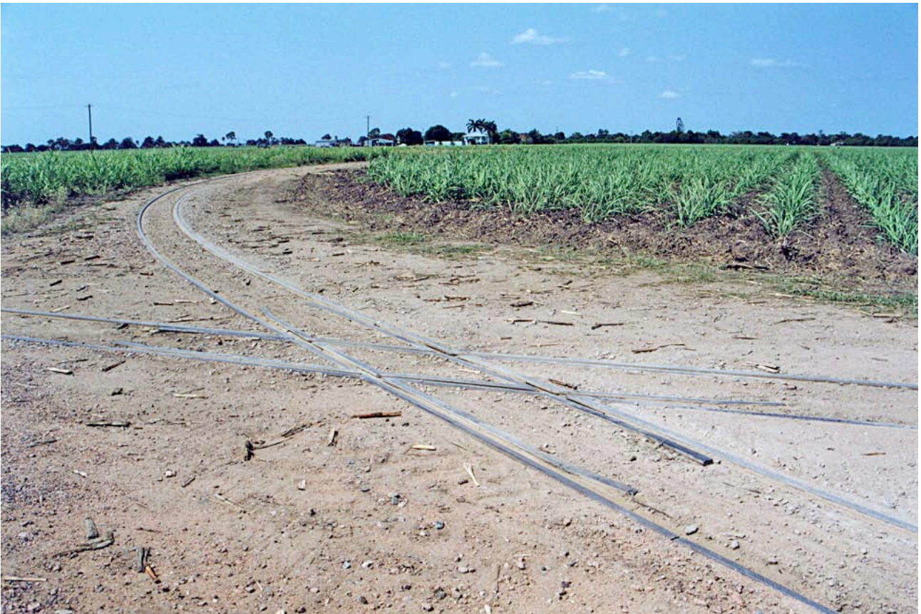
Diamond crossing on the Kalamia Mill system.
