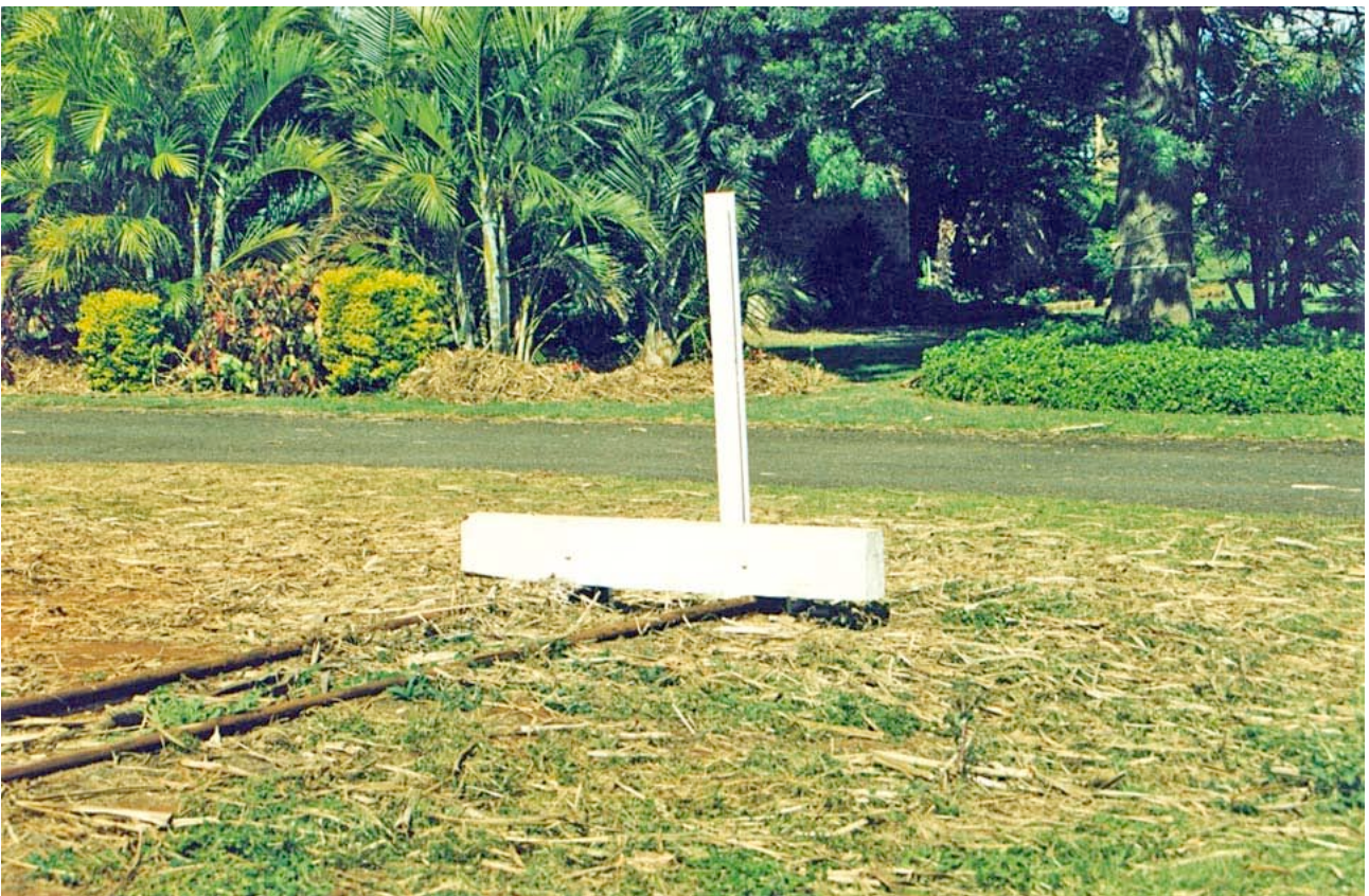
Rail and timber buffer
