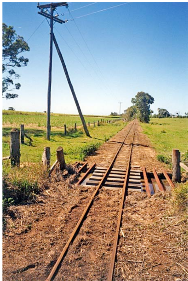
Basic rail and sleeper cattle guard constructed in situ. A more elaborate example is shown below.
