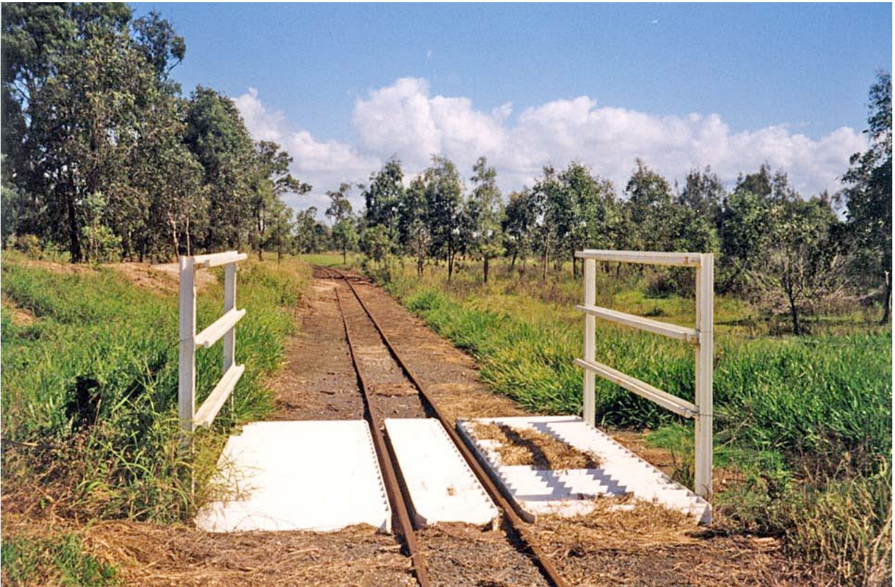
Cattle guard constructed from dimension timber
