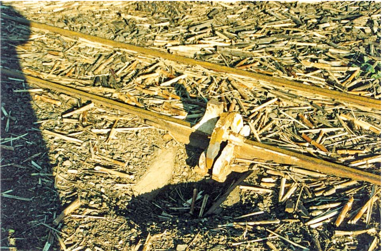
A siding on Bingera Mill's system that has both types of choke block at the one location.
