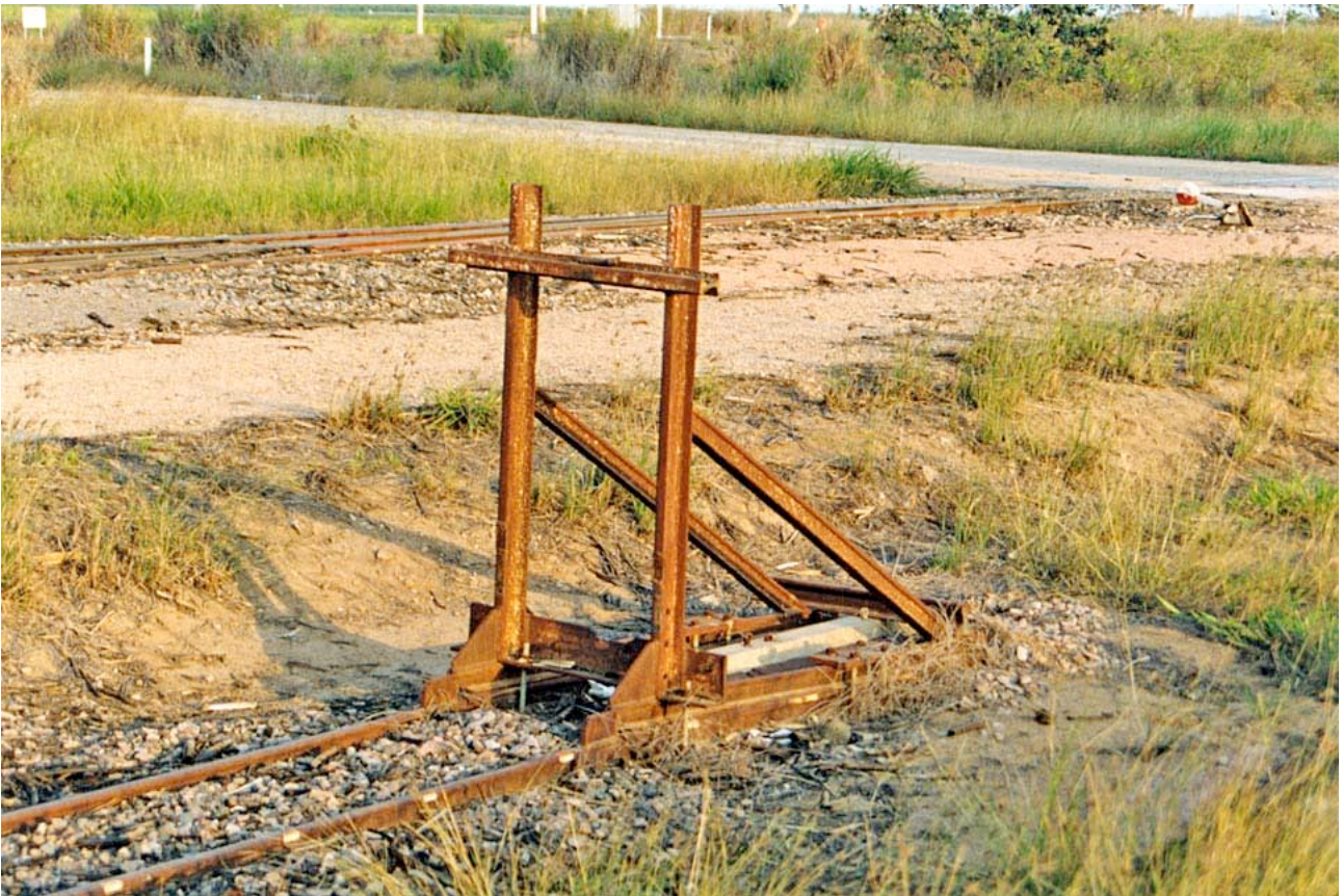
Fabricated rail buffer
